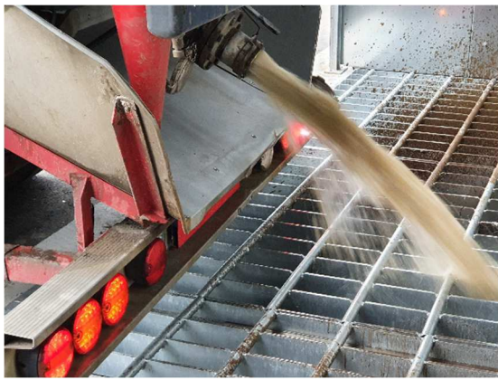
Emptying drilling fluid (liquid phase) from vehicle
