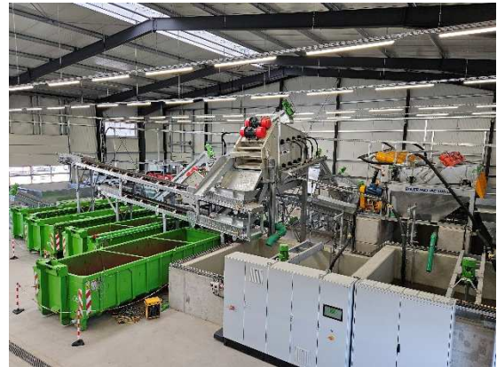
Recycling plant with containers for mineral fractions
