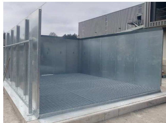
Feeding hopper for emptying/ cleaning the vehicles
