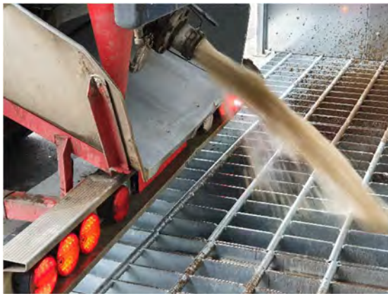
Emptying drilling fluid from silo vehicle
