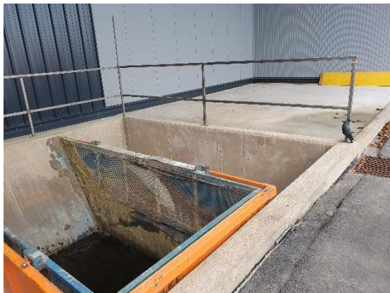
Initial situation: Existing concrete basin at customer's site
