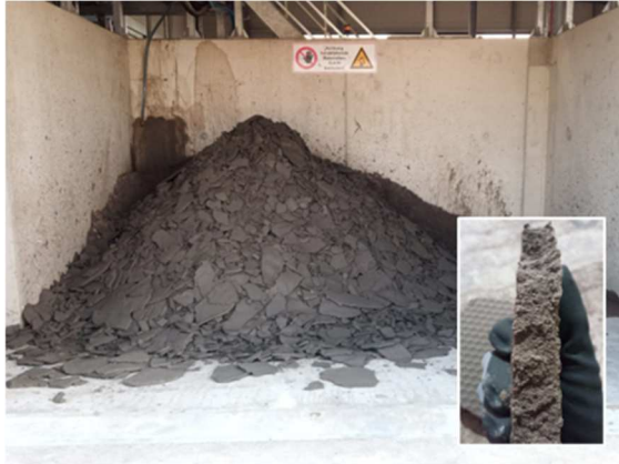
Filter cake from recycling of bentonite suspension
