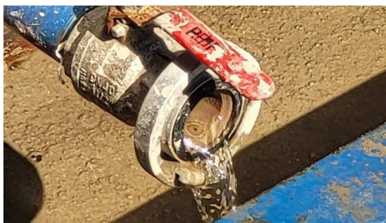
Filtrate discharge dewatering container
